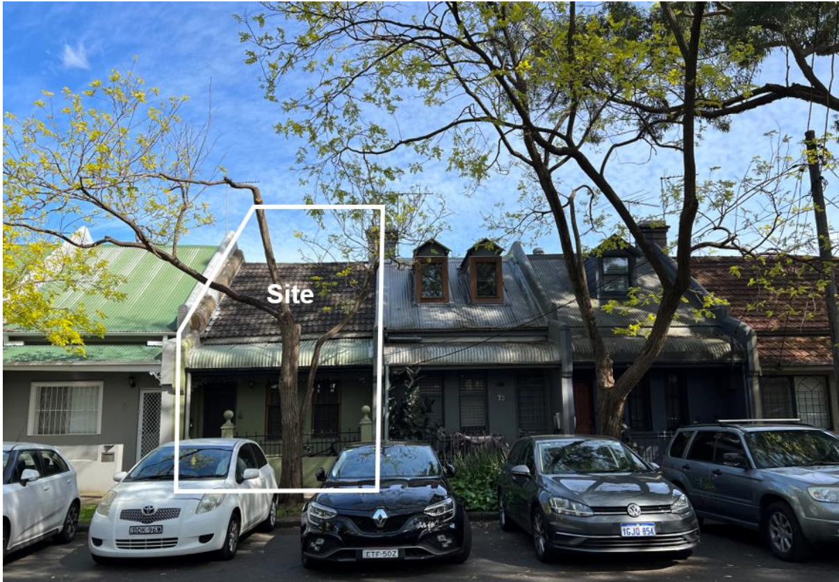
Figure 2: Site viewed from Kepos Street, and adjoining 71 and 73 Kepos to the right
