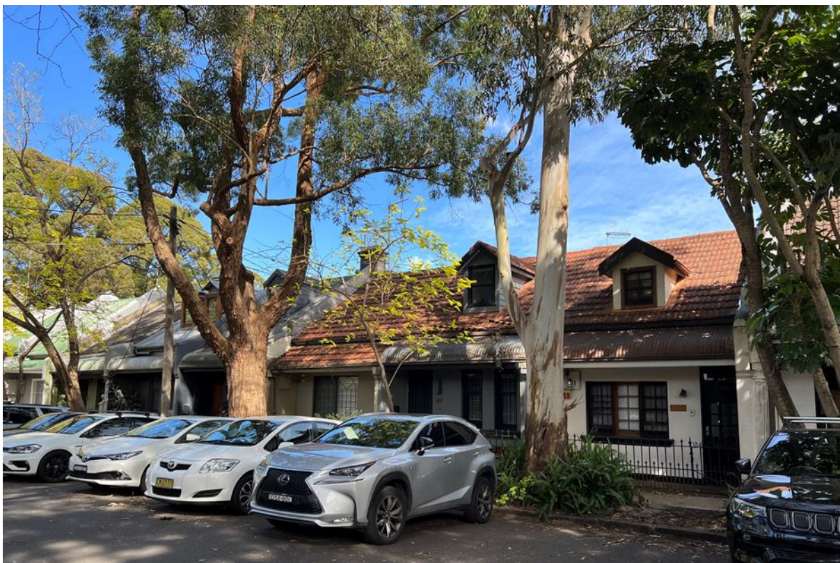
Figure 3: Neighbouring terraces further to the north, viewed from Kepos Street
